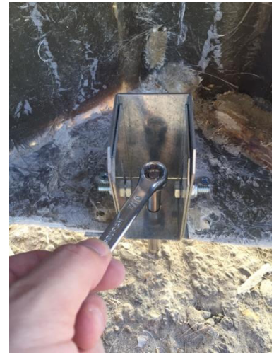
Place anchor and tighten
