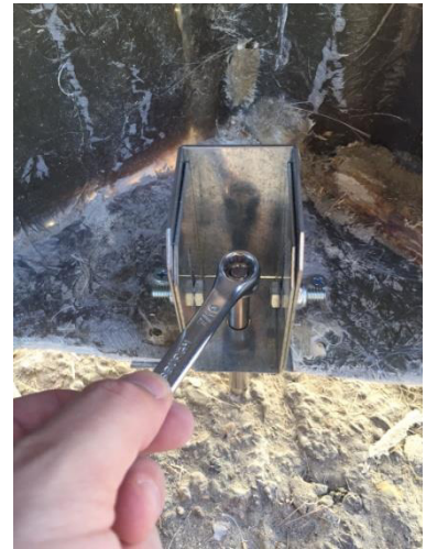
Place anchor and tighten
