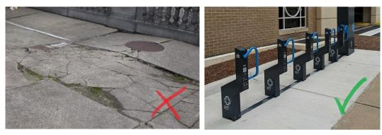
Docks bolted to the ground with a new concrete surface creation (Type 2)
